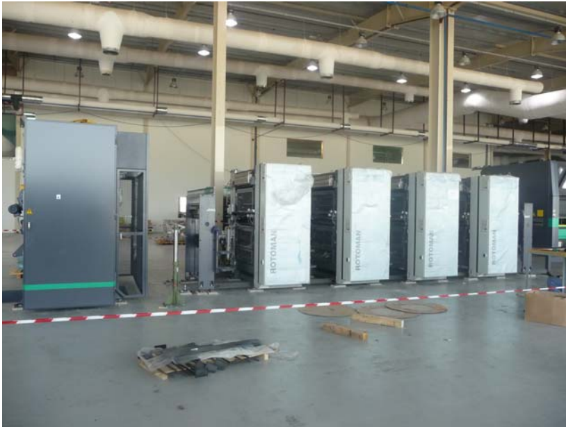
The Rotoman 65 while under commissioning a few months ago
